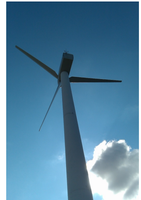
Vestas V27 225kW WT located at Sopko site
