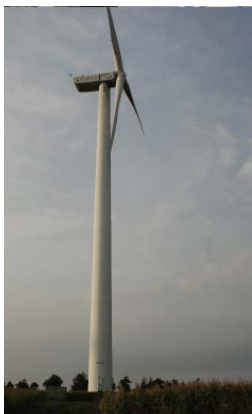
Nordex N54 1.0MW WT located at Sopko site
